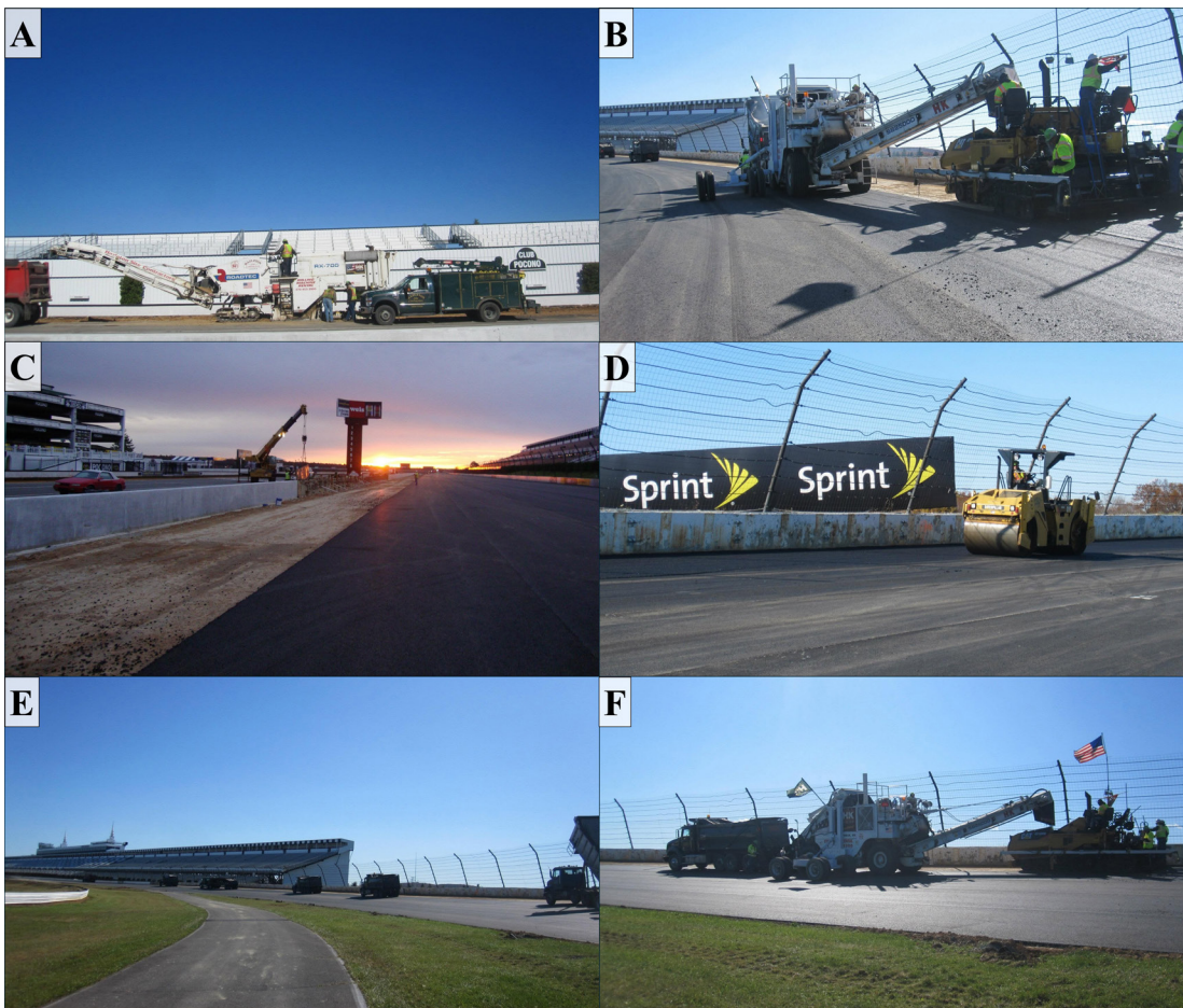
Figure 9. Photographs of the 2011-2012 repave project at the Pocono Raceway including a) removal from the existing wearing surface down to the dirt foundation and b-f) re-pave using the blast furnace slag asphalt mixture. Source: Pocono Raceway Facebook page Track Improvement photo album.
