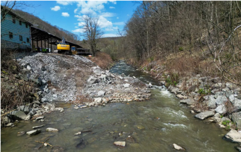
Figure 5.3. Photograph of Toby Creek mine subsidence work. Note: Photograph by J. Ardan, 2024. From “Water flow restored to Toby Creek in Luzerne after mine subsidence,” by S. Mocarsky, 2024, Wilkes-Barre Citizens’ Voice , https://www.citizensvoice.com/2024/04/15/water-flow-restored-to-toby-creek-in-luzerne-after-mine-subsidence/ . Copyright 2026 by Wilkes-Barre Citizens’ Voice.
