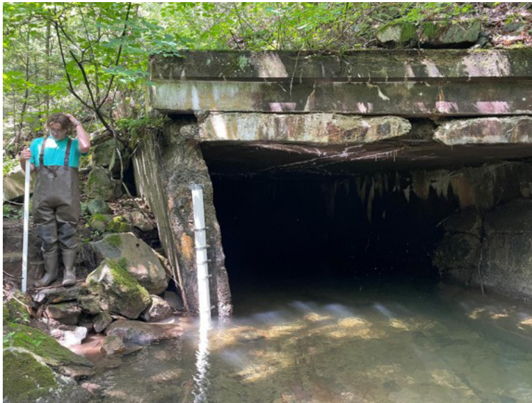
Figure 3. Photograph of the stilling well and gauging station installed on Laurel Run for continuous measurements of stage (water levels) and temperatures at 5-minute intervals.
