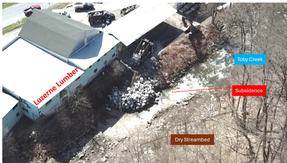
Figure 5.2. Mine subsidence and emergency remediation at Toby Creek on April 14, 2024. Note: Screenshot captured from the WNEP-TV news video Mine subsidence in Luzerne County (Kohut & Strub, 2024).
